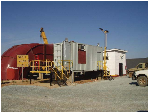
Mobile electric room for exhaust fans
